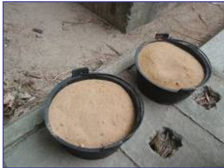
Excavated materials during construction
